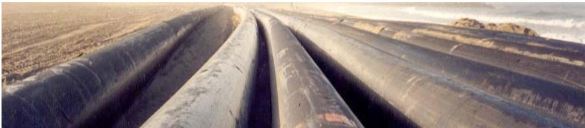
The nature of this structure can be seen as a manifold that can be filled with air, sand slurry, or concrete for ballast at different times during construction and deployment. When filled with air (immediately after construction) the reef can be towed into position and then “sunk” and anchored to the ocean floor.
